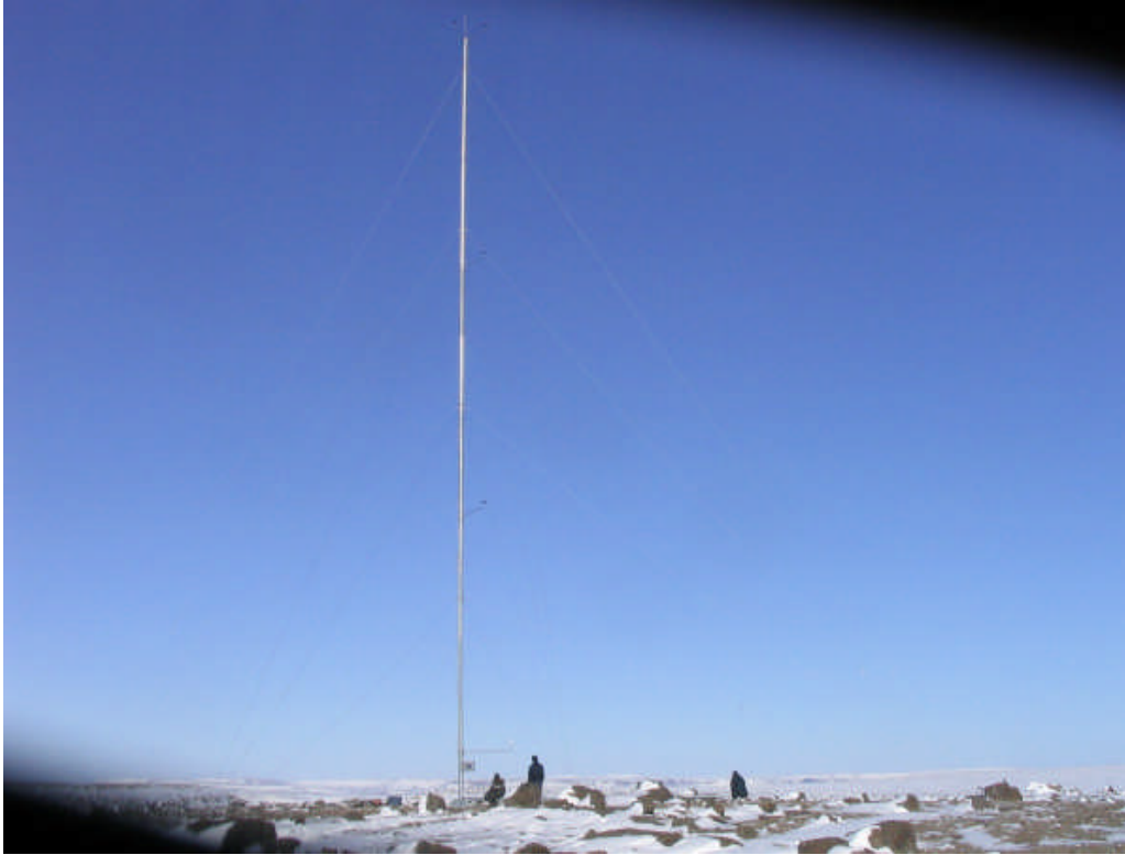
Figure 1: View of the wind monitoring station facing towards the south-southeast.
