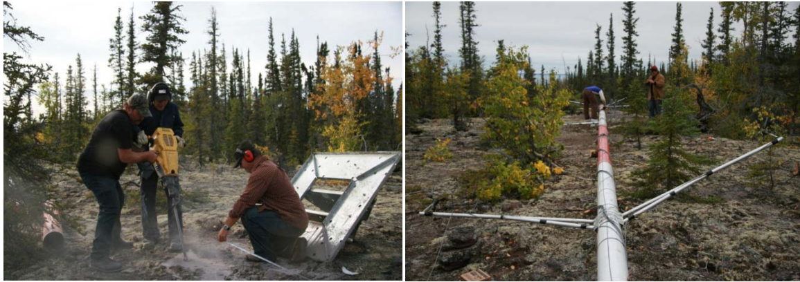
Figure 1: Installation of the wind monitoring tower near Hearne Channel, NWT.
