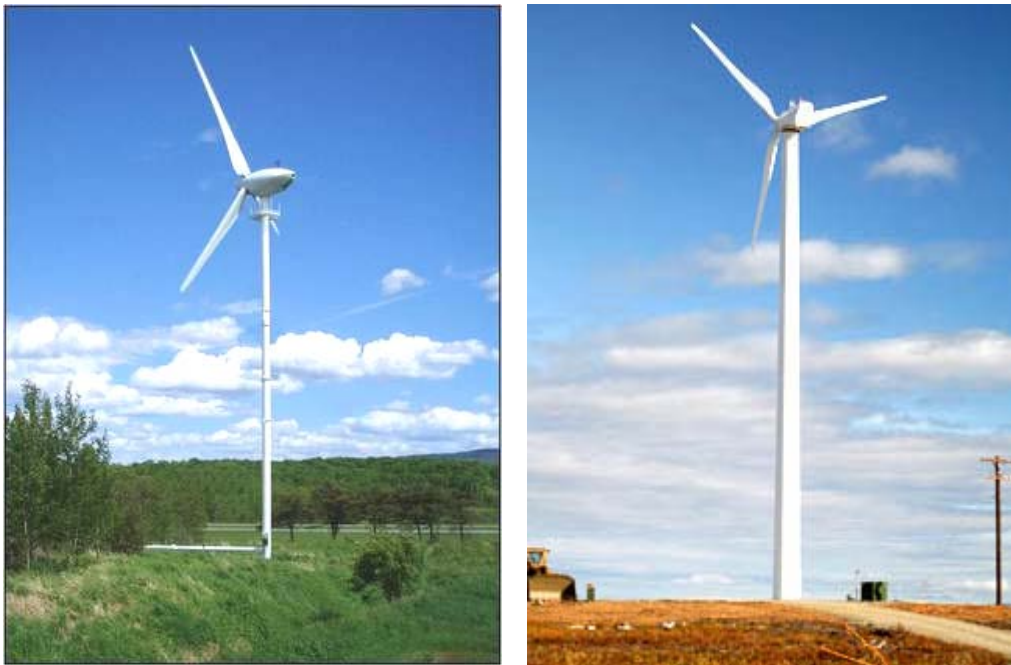
Figure 3: Two of the four wind turbines considered in the economic study for Lutselk'e. On the left is the Endurance E-3120 (55 kW) and on the right is the NorthWind 100 (100 kW).
