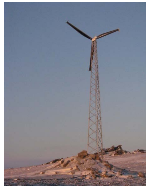
Figure 8: A EW50 wind turbine installed at Nome Alaska. This model is recommended for Ulukhaktok.
