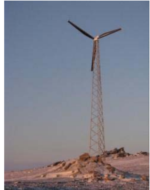
Figure 6: A EW50 wind turbine installed at Nome Alaska. This model is recommended for Sachs Harbour
