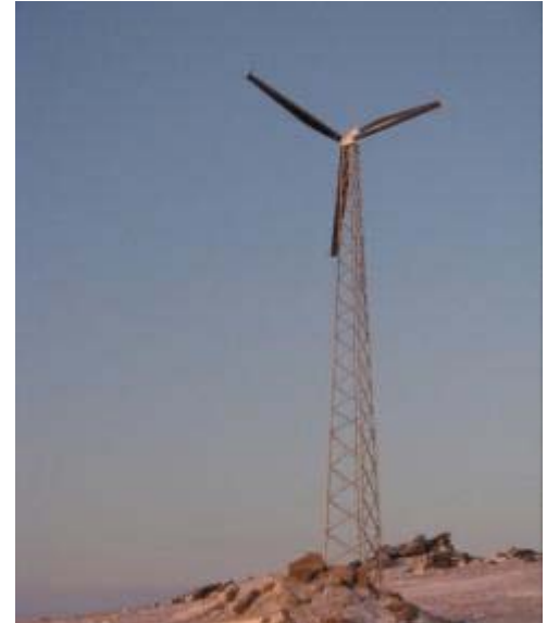
Figure 6: A EW50 wind turbine installed at Nome Alaska. This model is recommended for Paulatuk.
